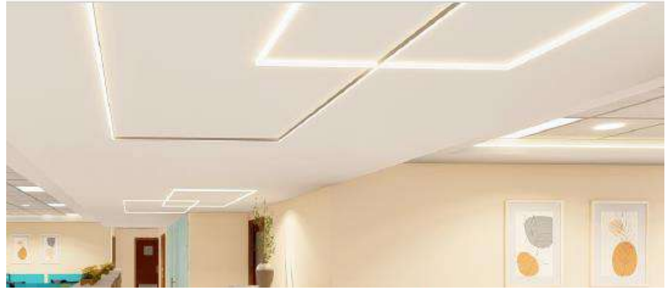
Grid And Gypsum Ceiling With 2'x2' Led Light Fixtures And LED Profile Light For General Office Area And Passage
