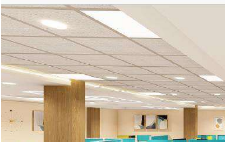
Grid And Gypsum Ceiling With 2'x2' Led Light Fixtures And LED Profile Light For General Office Area And Passage
